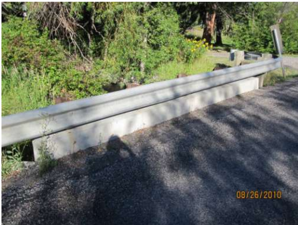
Photograph 6. Example of Curb on Bridge – Sourdough Creek
