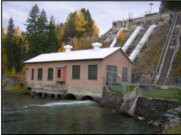
Figure 19. Bigfork Power House.
