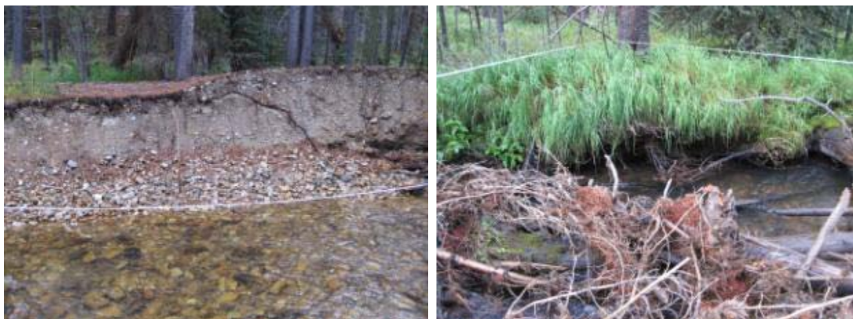
Figure 4-1. Typical eroding streambank conditions in Basin Creek Reach 08-02.
