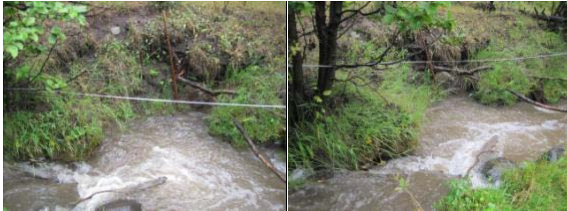
Figure 4-13. Typical eroding streambank conditions in High Ore Creek Reach 09-01.
