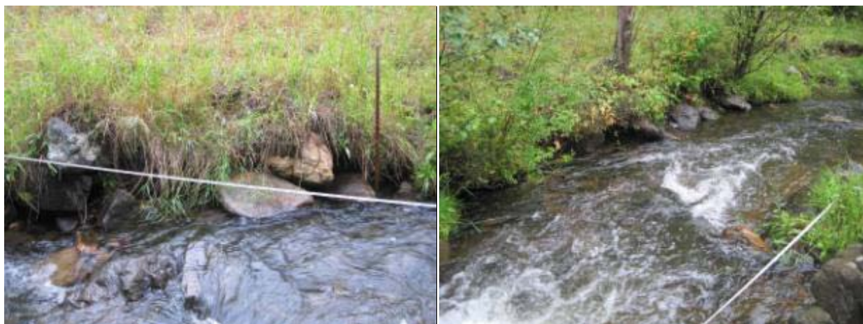
Figure 4-11. Typical eroding streambank conditions in Elkhorn Creek Reach 23-01.
