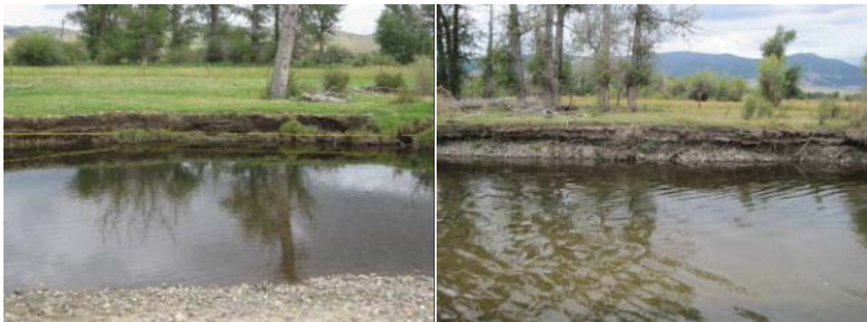
Figure 4-7. Typical eroding streambank conditions in Boulder River Reach 13-10.
