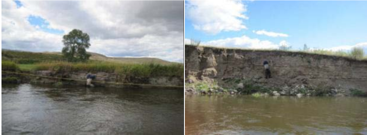
Figure 4-8. Typical eroding streambank conditions in Boulder River Reach 13-23.
