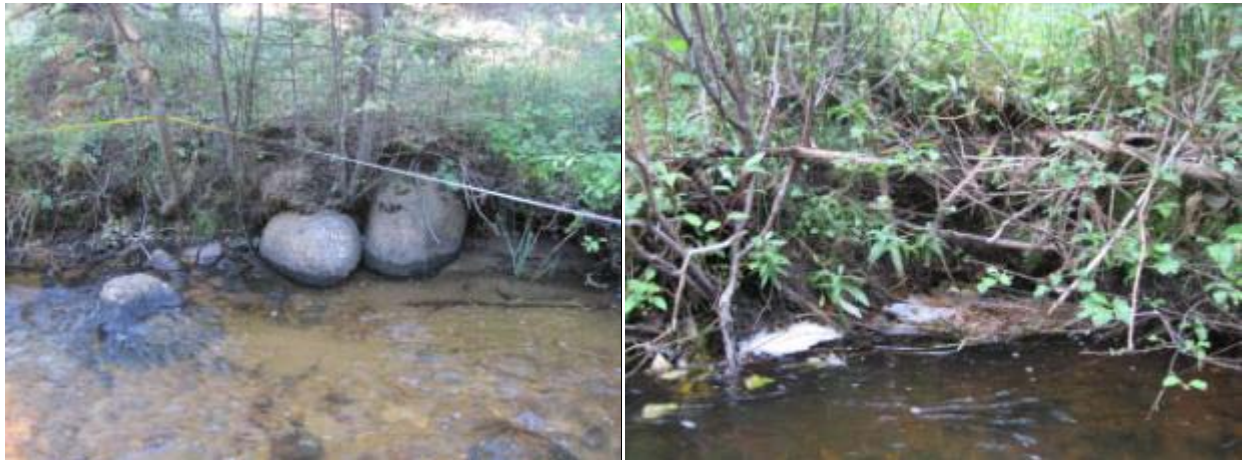
Figure 4-15. Typical eroding streambank conditions in Little Boulder River Reach 32-01.
