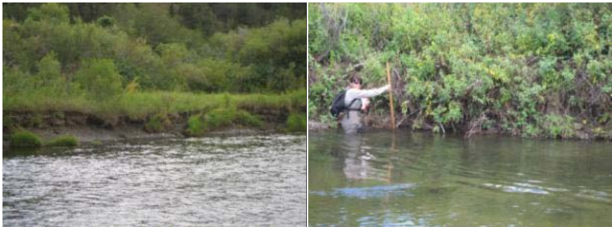
Figure 4-9. Typical eroding streambank conditions in Boulder River Reach 13-33.
