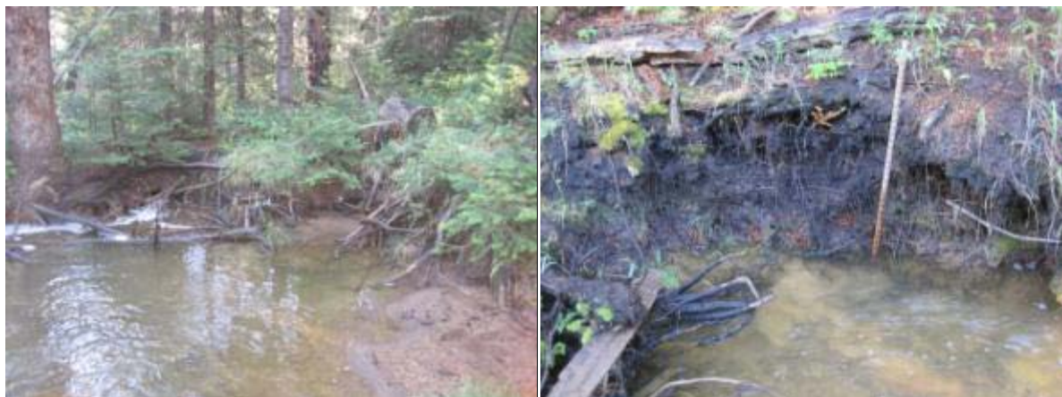
Figure 4-23. Typical eroding streambank conditions in Uncle Sam Gulch Reach 10-01.
