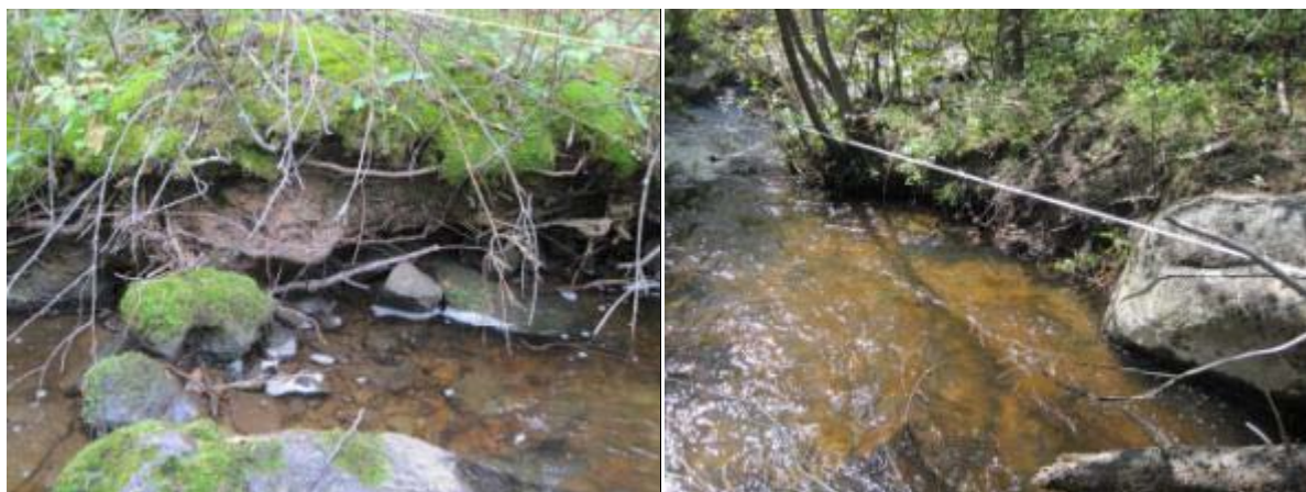
Figure 4-21. Typical eroding streambank conditions in North Fork Little Boulder 42-01.
