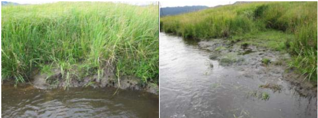
Figure 4-20. Typical eroding streambank conditions in Muskrat Creek Reach 22-08.
