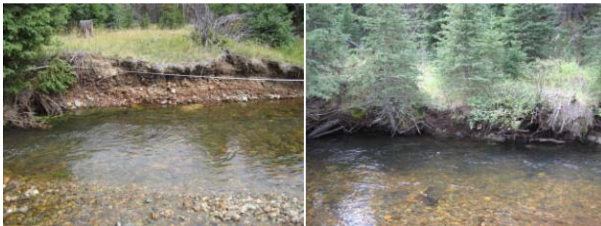
Figure 4-2. Typical eroding streambank conditions in Basin Creek Reach 15-02.
