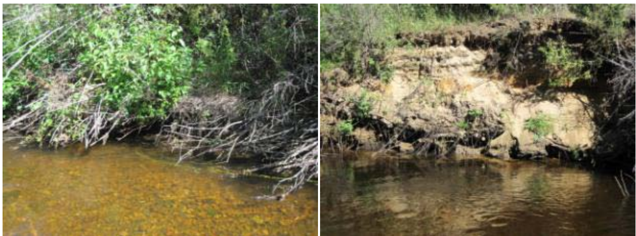
Figure 4-16. Typical eroding streambank conditions in Little Boulder River Reach 37-01.
