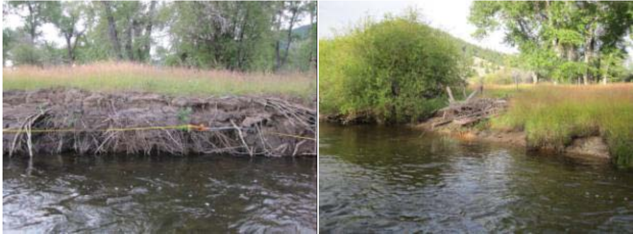
Figure 4-6. Typical eroding streambank conditions in Boulder River Reach 13-04.
