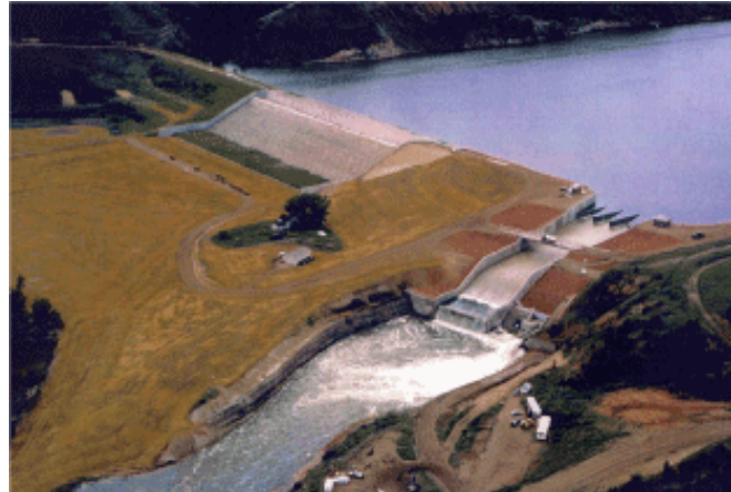
Tongue River Reservoir and Dam. Photo by Montana DNRC
