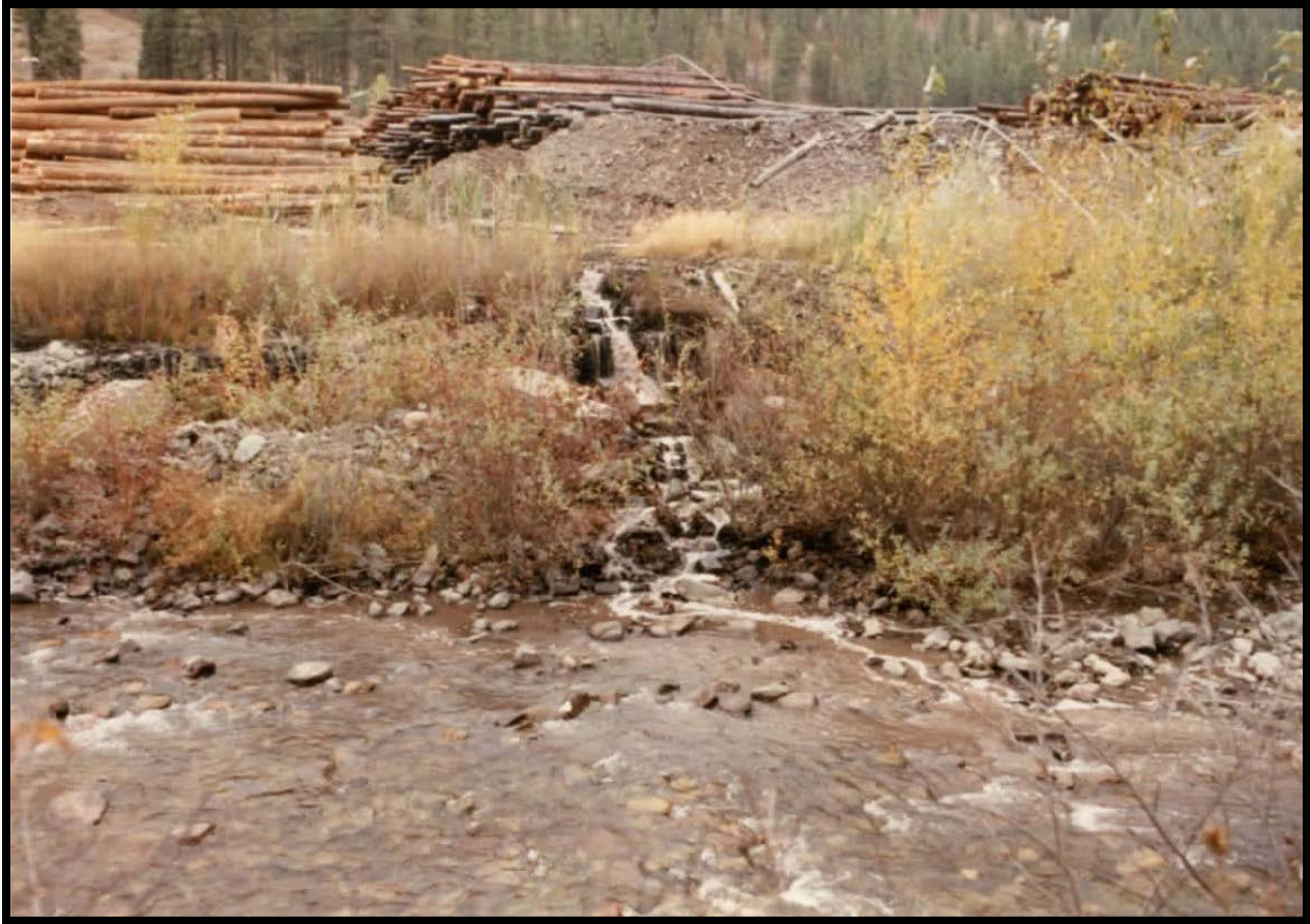
Figure 8-4. Photo T-2 of surface water discharge from log pond to Trout Creek, 10/3/1990.
